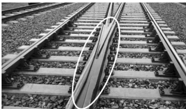
Fig. 1. Monoblock frog of high-manganese austenitic cast steel [L. 5]
